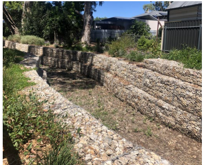
Rock filled gabions
