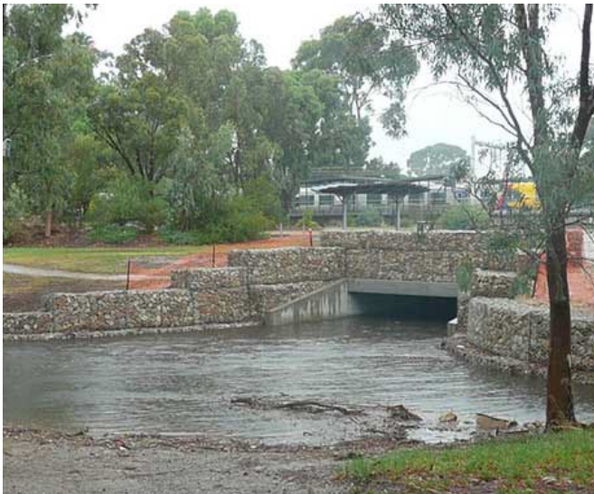
Constructed Culvert
