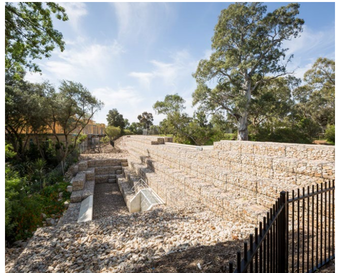
Flood Control Dam
