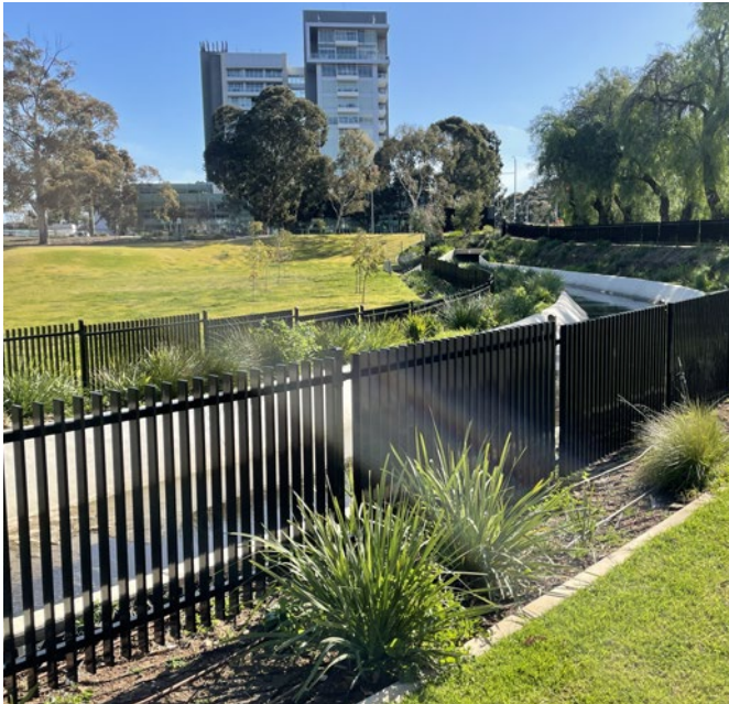
Concrete swale and fencing
